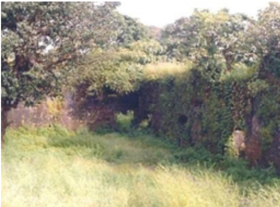
Fig. 3 wilderness growth (left) and Fig. 4 creepers penetrating walls (right) fort before restoration: (Academy of Architecture Mumbai)
