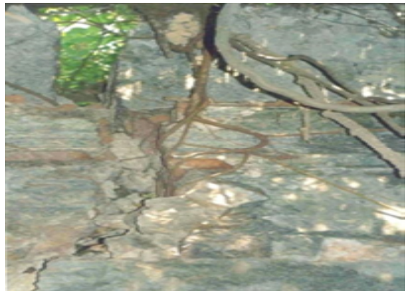
Fig. 3 wilderness growth (left) and Fig. 4 creepers penetrating walls (right) fort before restoration: (Academy of Architecture Mumbai)
